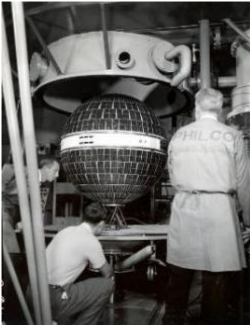
Courier 1B; world's first active repeater satellite. Launched in 1960.
